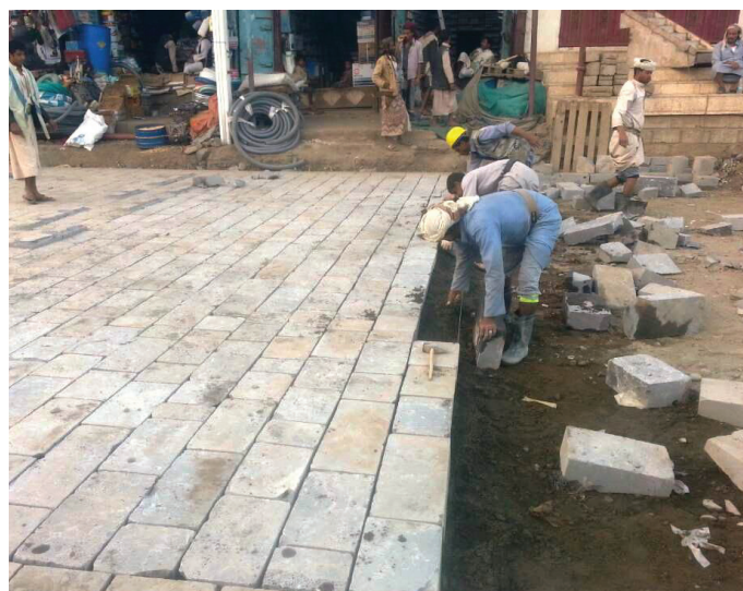
Employing the poor in paving Al Qafra Souq in Amran
