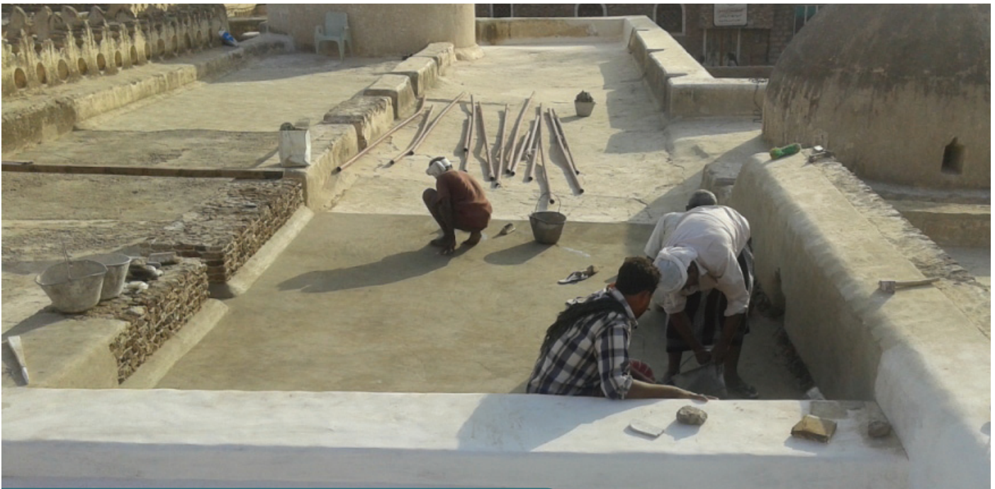
Rehabilitating part of roof of Alasha'er mosque in Alhodeida
